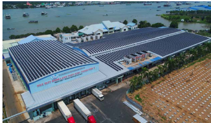
Sao Mai Group, Dong Thap 1,0160 kWp (2017)
