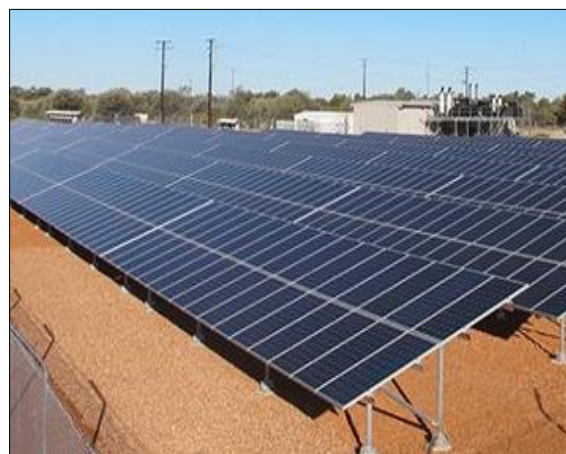
Image 5 (Mini-grid photovoltaic system with ESS)
